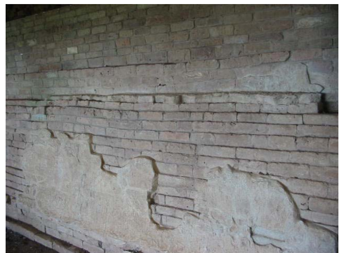
Figure 16. Ancient brickwork of Jetavan Stupa
