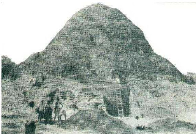
Figure 19. Miriseveti stupa after an unsuccessful restoration attempt
